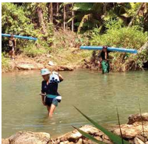
Construction of new water pipe system
